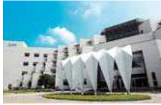
Tainan Plant (Diamond-rated Green Building)
